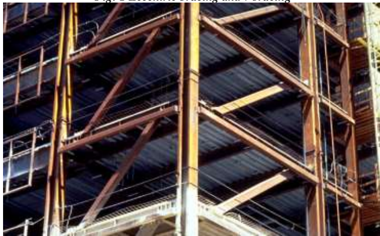
Fig: 2 Eccentric bracing in structure
